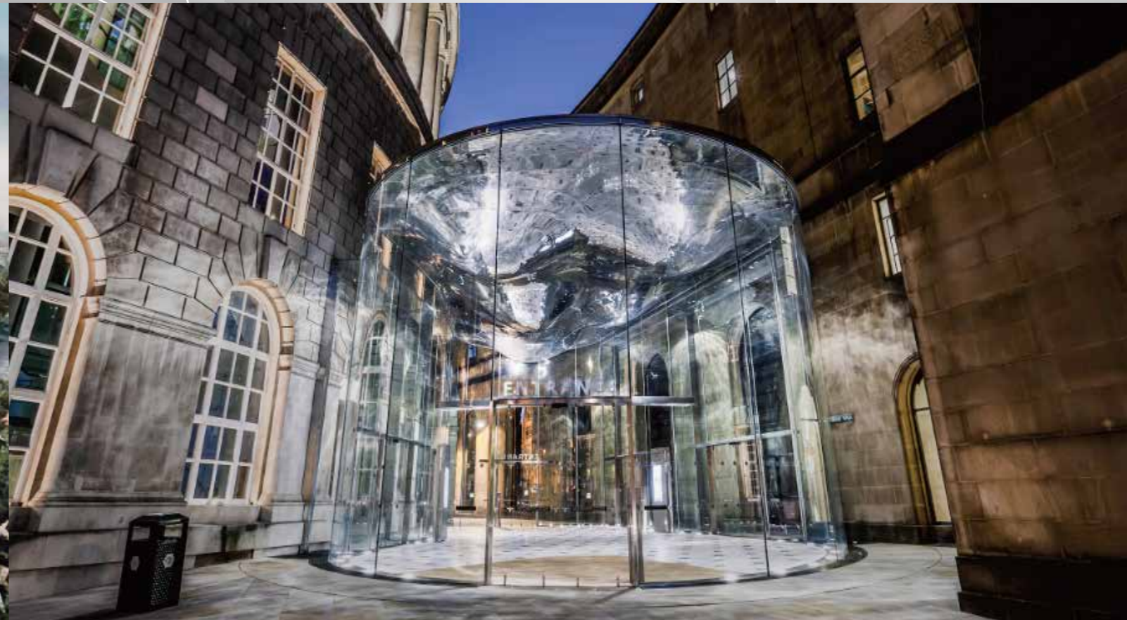
▲ Manchester Town Hall, UK Glass makeup: 3×12mm low iron glass curved tempered HST+2×1.52 SGP Furnace used: AC15E128
