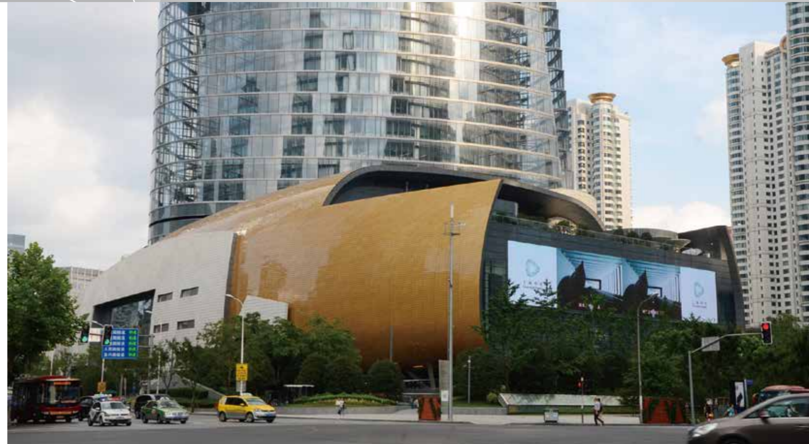
▲ Shanghai Tower Glass makeup: 6mm Glazed glass HS +1.52PVB + 6mm Solar control coated glass (4#) +16 AR + 6mm Clear glass + 0.38PVB + 6mm Clear glass Furnace used: B22S2536 & B15B8050
