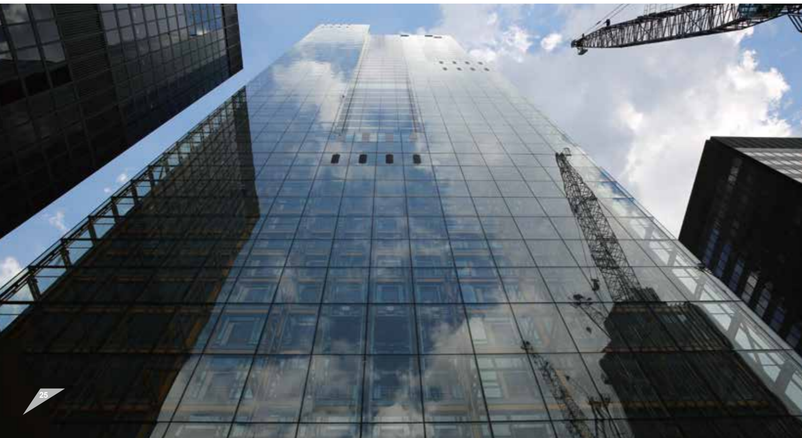
▼ London Leiden Building, UK Glass makeup: 6mm glazed glass HS+1.52PVB+6mm SunGuard SN51/28 Low-E glass HS (4#) +16 AR + 6mm clear glass+0.38 PVB + 6mm Clear glass Furnace used: AD1B80-GUD
