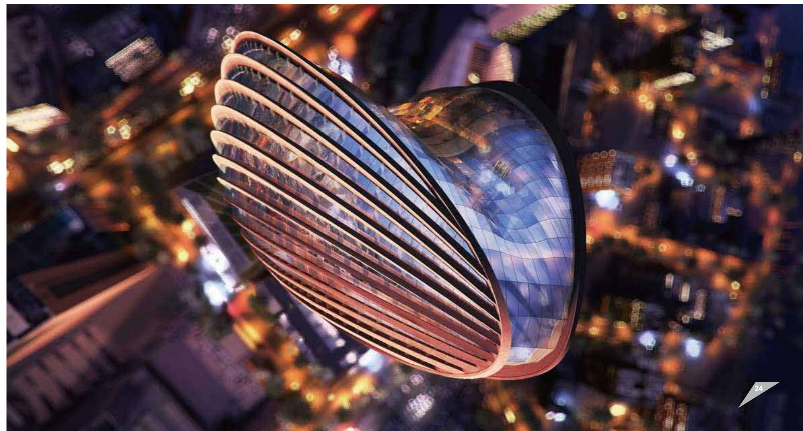
▼ National Bank of Kuwait Glass makeup: 8mm Heat-reflective glass+1.52PVB+8mm clear glass HS+16A +6mm double Ag Low-E glass 8mm Heat-reflective glass+1.52PVB+8mm clear glass Tempered+16A+6mm double Ag hLow-E glass+1.52PVB+6mm Tempered glass Furnace used: AG15B50 (bending upwards & downwards)
